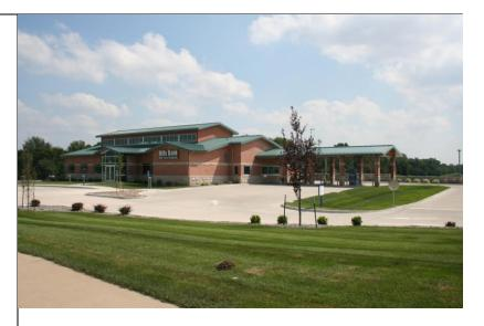
Constructed in the North River Village Development, on the Northeast side of Cedar Rapids, this new branch bank for Hills Bank & Trust incorporates a masonry façade of limestone, rose-velour brick, as well as green tinted glass, and a prefinished metal roof, as required by the restrictive covenants developed by AEGON for this development.
